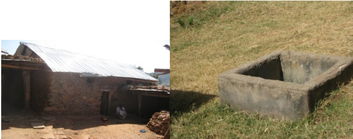
Cattle shed-left & right of the front house (left); and, biogas ingredients mixer (right)
