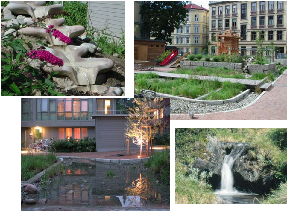
Fig. 2. The klosterenga greywater treatment system. Upper right; the wetland in the foreground the biofilter is underneath the playground behind the stonewall. Upper left; Flowforms. Lower left the effluent is exposed in a shallow pond. Discharge to a local stream is possible if the stream was reopened.
