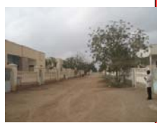
2. Concrete-constructed houses and buildings
